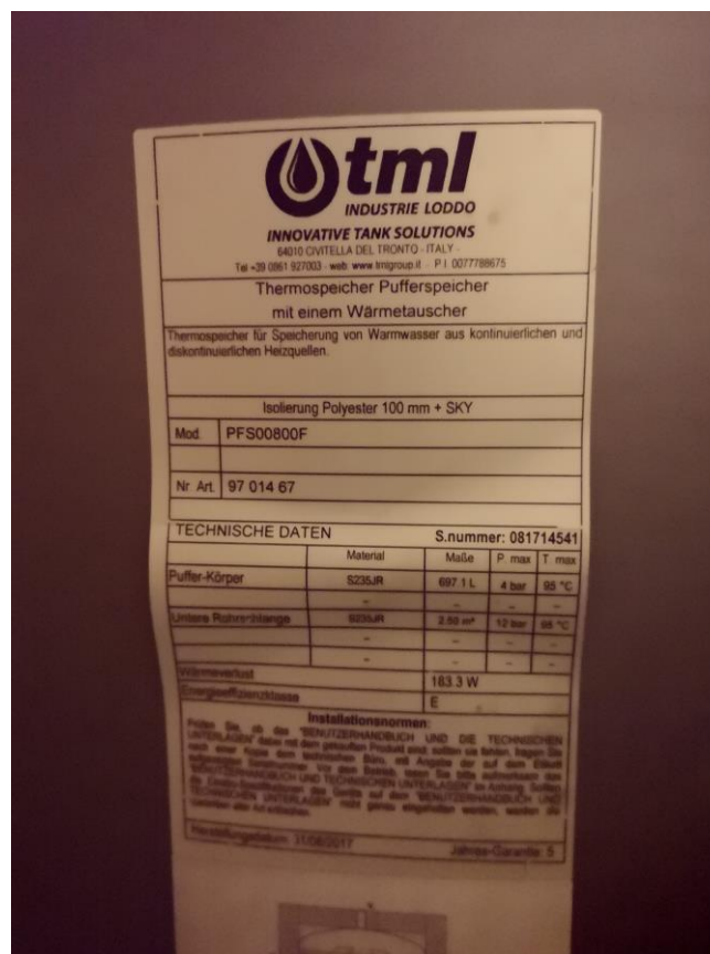
Figure 23: Space heating storage data plate
