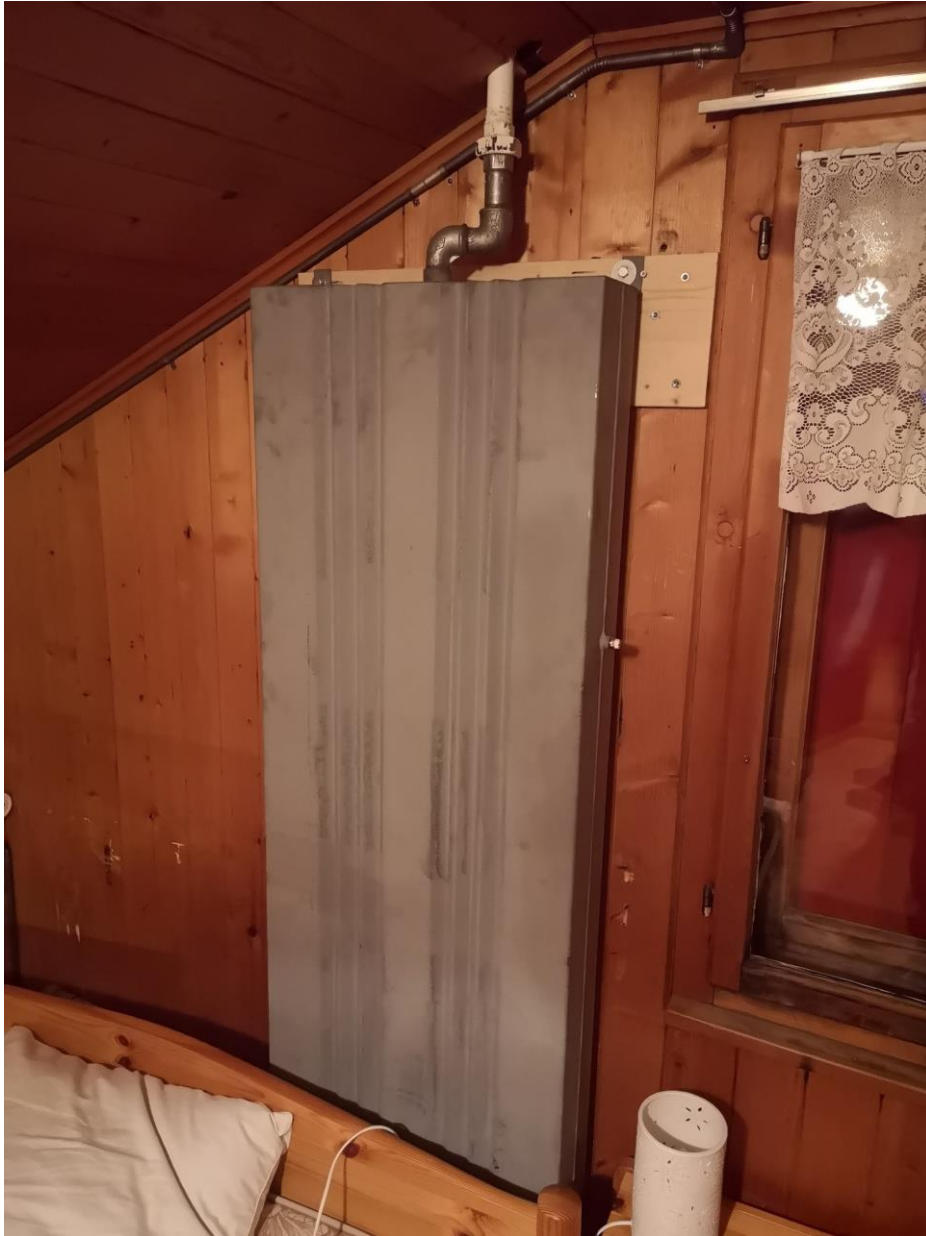
Figure 32: Expansion tank (top floor)
