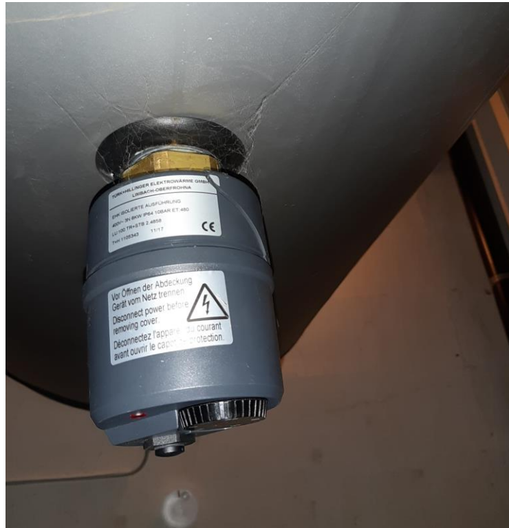
Figure 26: Immersion heater (space heater)
